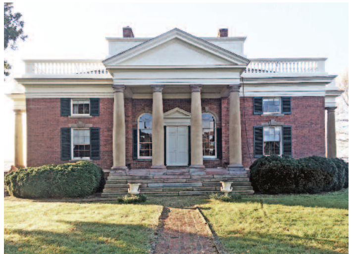
North Elevation of Bremo after restoration Photo by Gibson Worsham
