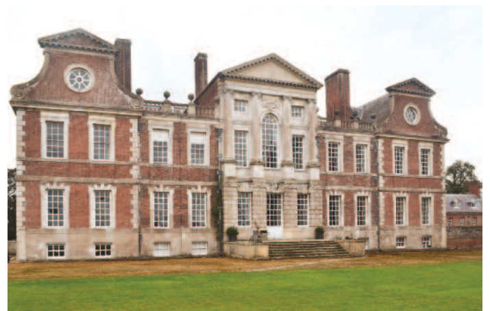
Raynham Hall, Norfolk Photo by Calder Loth
