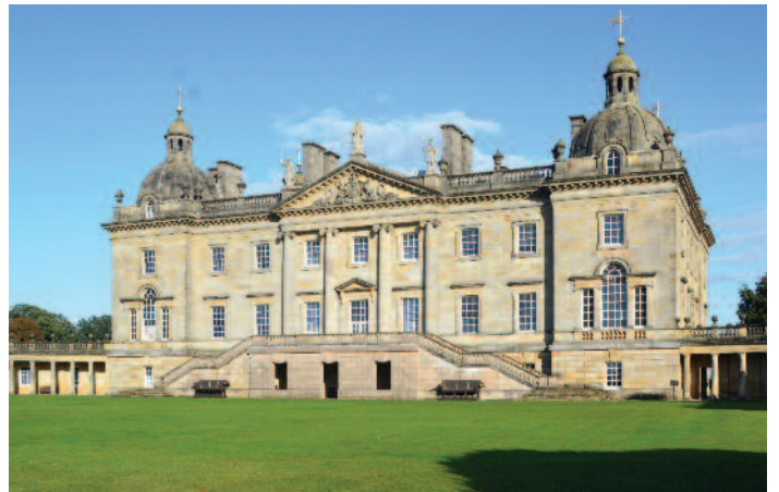
Houghton Hall, Norfolk Photo by Calder Loth
