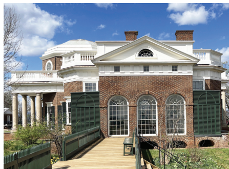
Southeast elevation of Monticello showing the metope windows and greenhouse Photograph by Noah Duell
