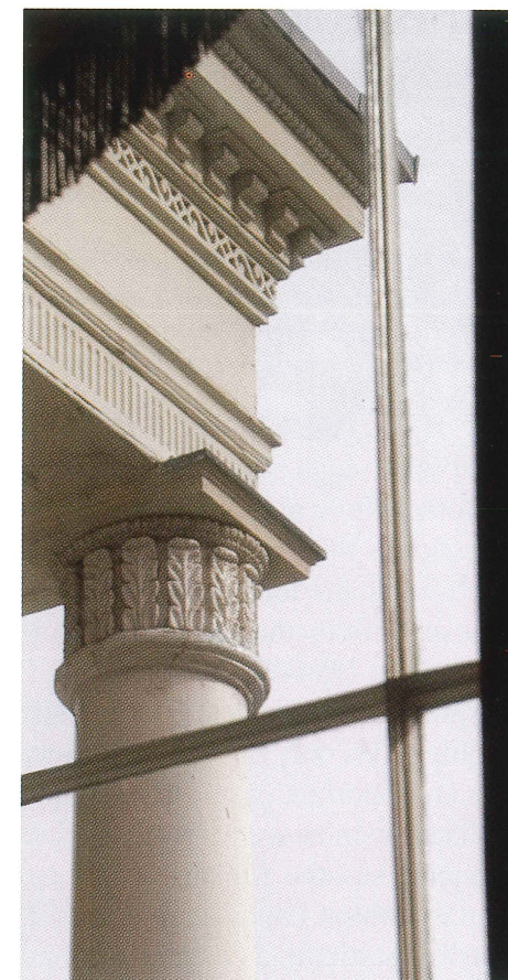
Fig.3. Column, capital and entablature of the portico at Homewood, from dining room.
