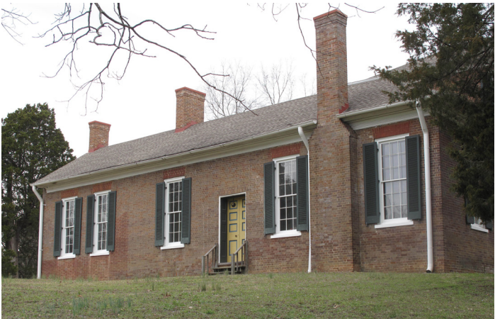
View of east wing looking southwest, with rubbed brick flat jack arches, polychrome door, and replaced brickwork dating to restoration Photograph by author
