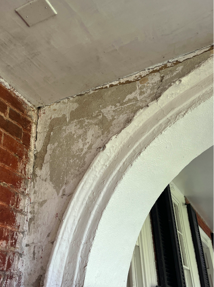
Pavilion VII, University of Virginia Exposed faux ashlar on inside corner Photograph by author
