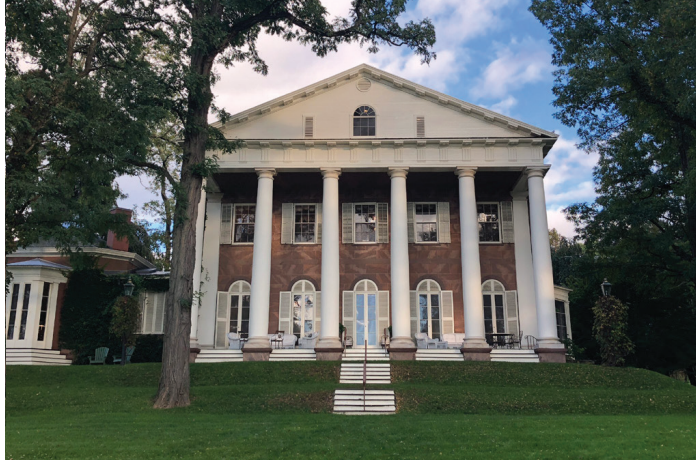
Edgewater, West Facade, Barrytown, NY
